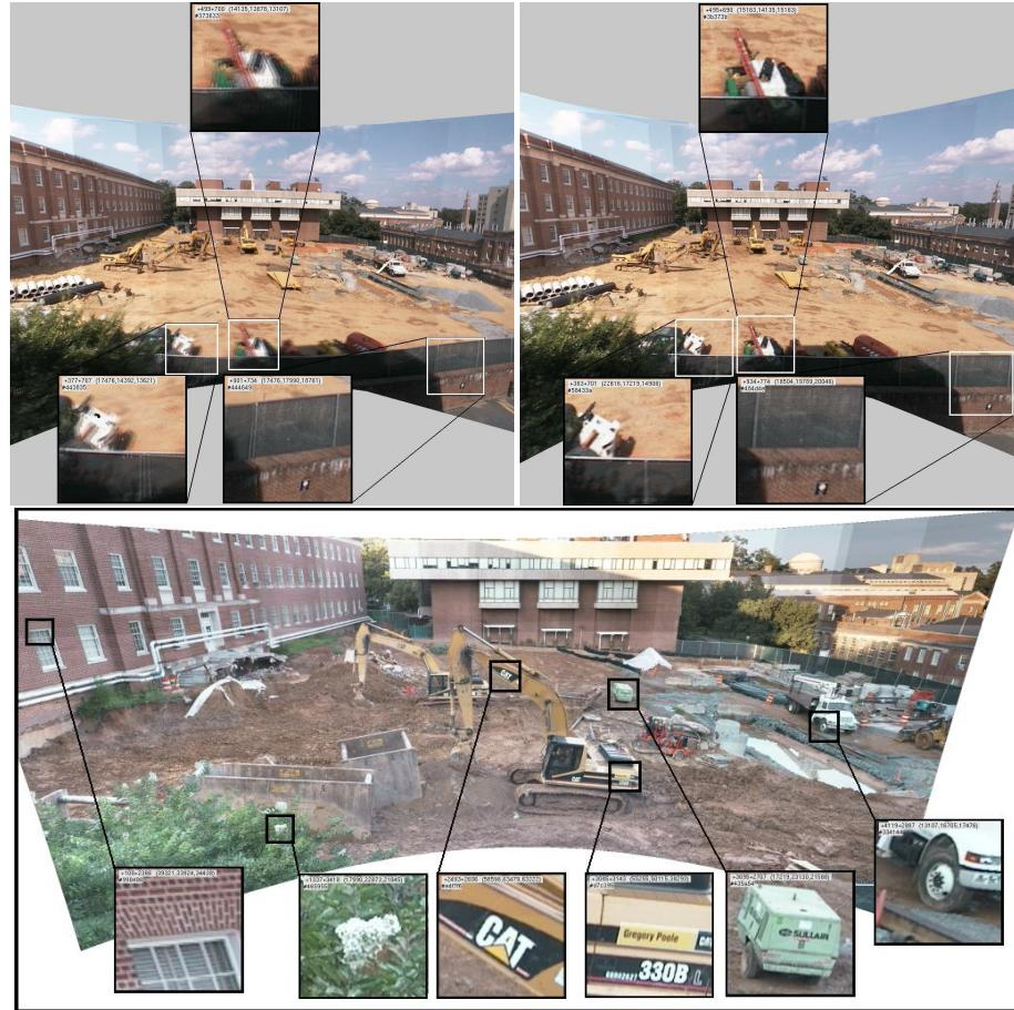
**Fig. 4.** The front face of the computed cube-maps: (a) Radial distortion was ignored in the camera model (Note that straight lines in the world are not imaged as straight lines). (b) Accurate panorama created after incorporating radial distortion. (c) High-resolution panorama ( $6000 \times 6000$  pixels) built from 119 images at 5X zoom. Note the zoomed-in regions of the panorama, displayed in the original scale.
