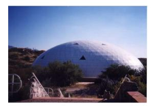
The two lungs are responsible for keeping the air pressure in the Biosphere 2 system constant. Heavy concrete ceilings are suspended from the dome of the lungs, sealing the inside atmosphere by flexible rubber flanges. When the temperature within Biosphere 2 increases, the pressure increases as well, pushing the ceilings up, until the pressure is again equalized by increasing the volume of Biosphere 2.
